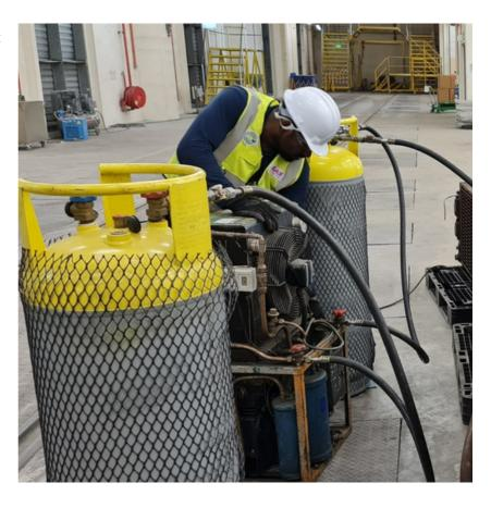
By recovering and reclaiming the R407C on behalf of the customer, A-Gas has initially abated 597 metric tons of CO2e, that otherwise may have been released into the atmosphere.
